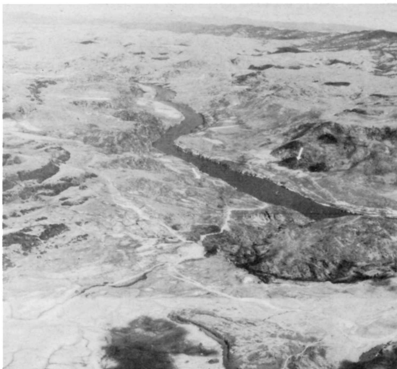
AERIAL SCENE FROM INSPIRATION POINT LOOKING NORTH DOWN RIVER, SHOWING MOUTH OF COULEE IN LOWER LEFT. THIS PICTURE WAS TAKEN BEFORE DAM CONSTRUCTION WAS STARTED. NOTE ARROWS SHOWING LOCATION OF DAM.
