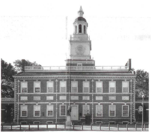
Independence Hall (A World Heritage Site)
