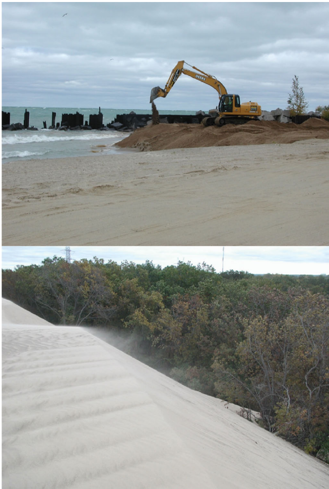
Figure 7. Photographs of issues associated with Mount Baldy. Coastal engineering structures interrupted the sand supply to Mount Baldy. This caused coastal erosion, which is under constant management to renourish the supply. Mount Baldy is now migrating inland, burying forests and threatening park infrastructure. National Park Service photographs taken in 2010.
