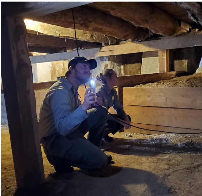
Park staff look at the logs in the basement of the Bauvais-Amoureux house. Researchers used the logs to date the house.
