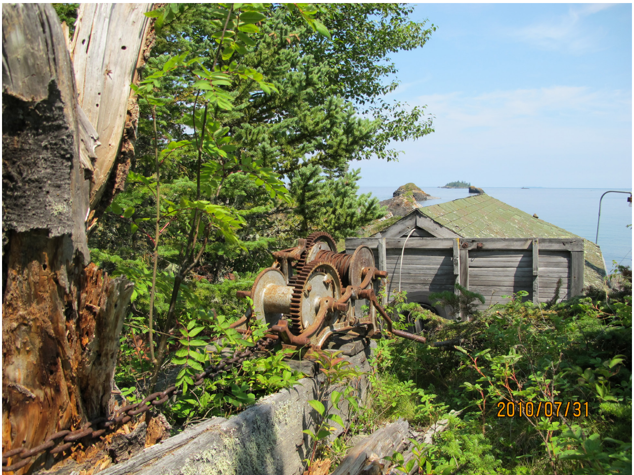
Winch to the rear of the boat house (Shafer/NPS 2010).
