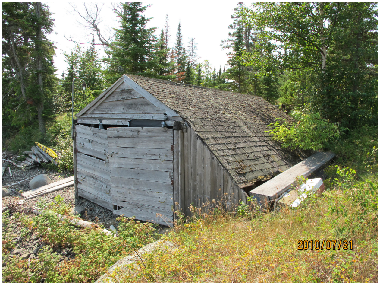
McPherren Boat House (Shafer/NPS 2010).
