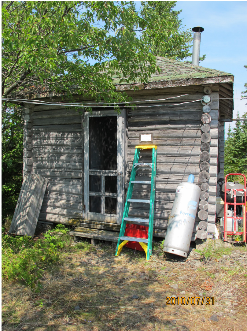
McPherren Bath House (Shafer/NPS 2010).
