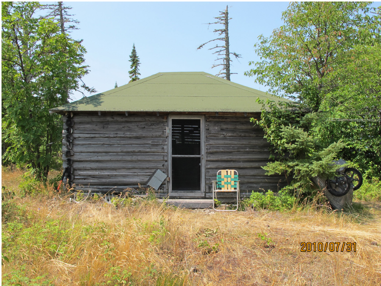
Sleeping Cabin III (Shafer/NPS 2010).
