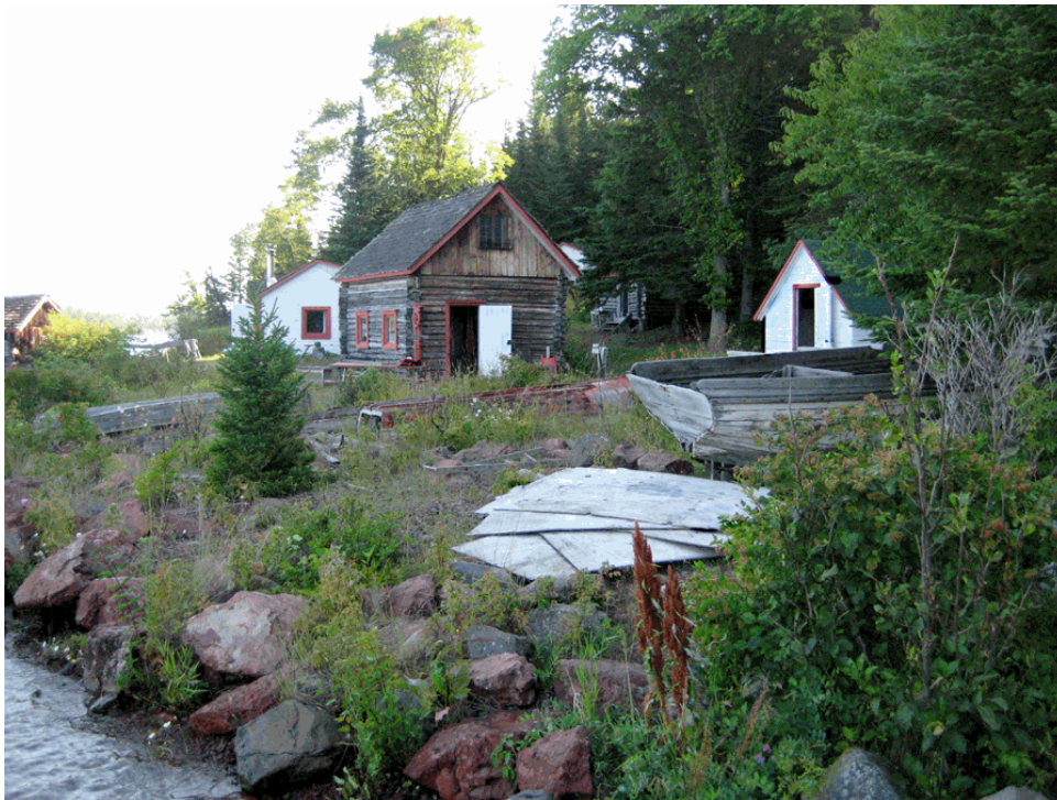
Edisen Fishery viewed from the concrete dock. (Hauser for NPS 2008)
