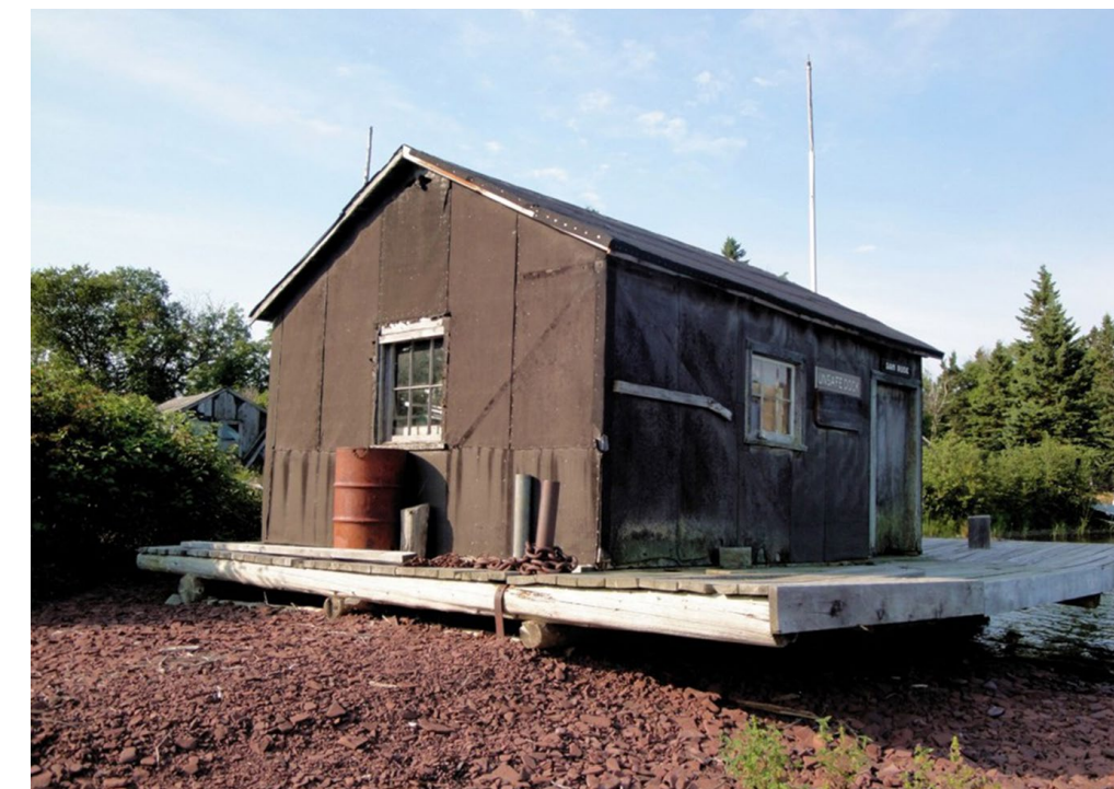
The Rude Fish House. Above, viiewed from the lake towards the shore, ca 1940 (NPS ISRO Archives). Below, viewed towards the lake from the shore, 2010 (Jackson/NPS)
