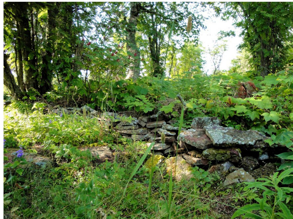
Dry-Laid Stone Wall (Jackson/NPS 2010)
