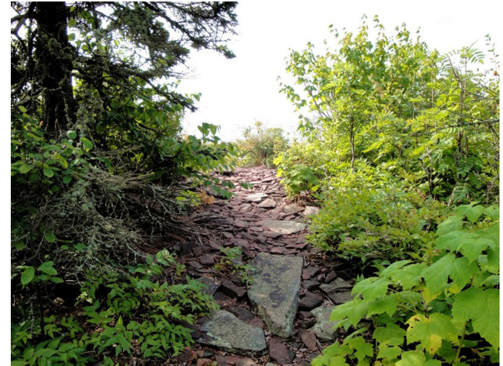
Stone walkway leading to the Lake Superior shoreline (Jackson/NPS 2010)
