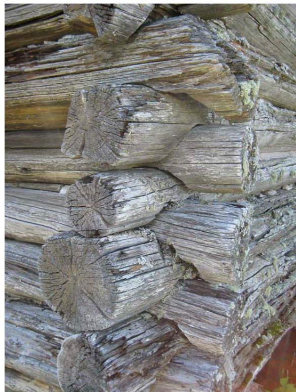
Saddle notching detail (NPS 2008)
