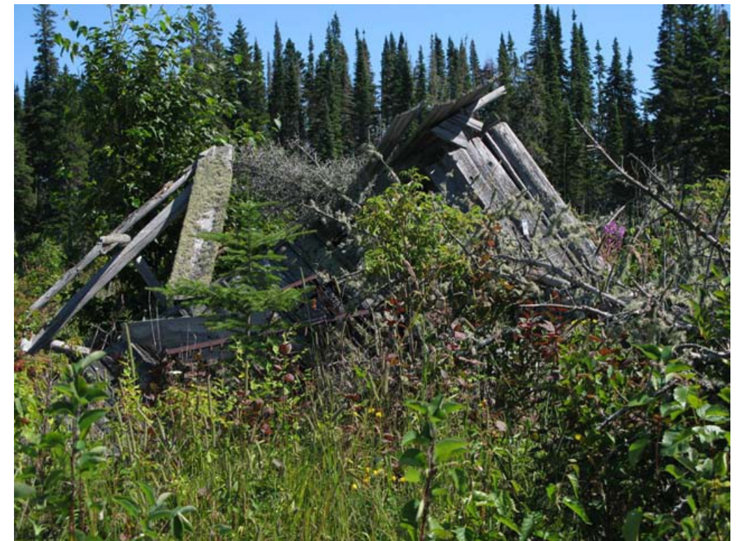
Net House ruins, facing south (NPS 2008)
