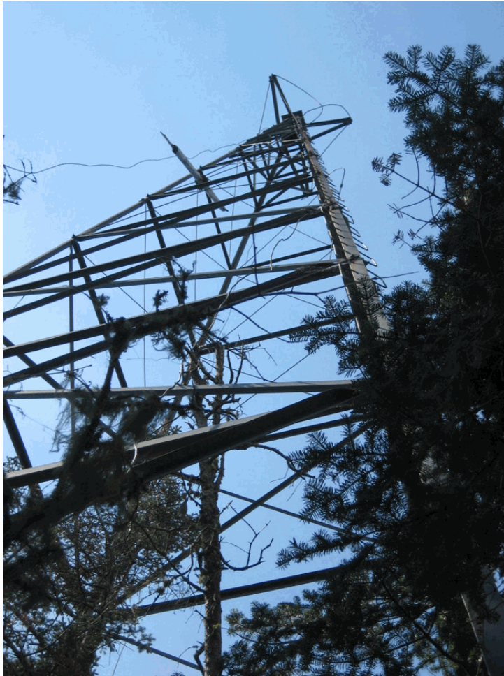
Radio Tower (#186C). (Gladstone for NPS, 2008)
