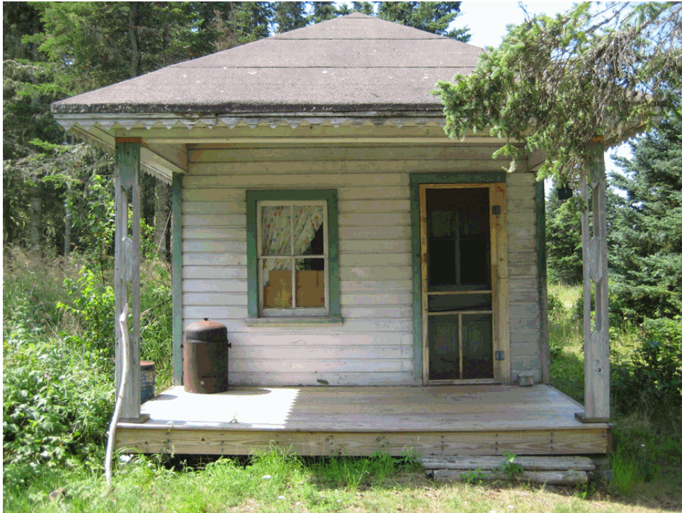
Honeymoon Cottage (#192). (Hauser for NPS, 2008)
