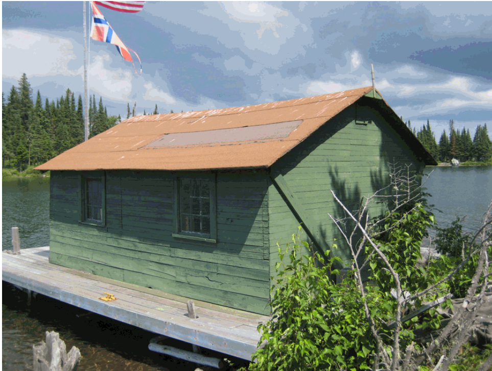
Ekmark/Eckel Fish House (#197). (Hauser for NPS, 2008)
