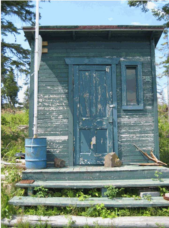
Sivertson Laundry (#194). (Hauser for NPS, 2008)
