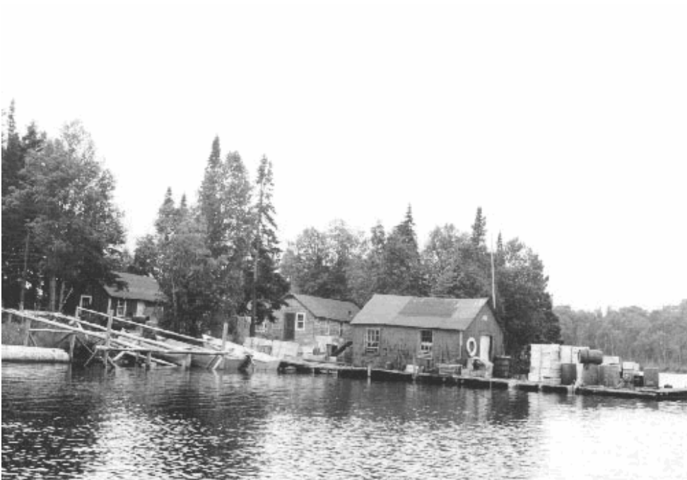
View of Washington Fishery. Fish House (#198), S. Sivertson Residence (#200), and Net House (#199). NPS file photo.
