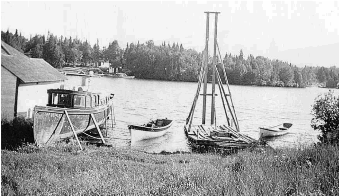
A view of Washington Island from Barnum Island, ca. 1930. The pound scow, center, was used to drive pound net stakes into the lake bottom. (Gale, 1995)
