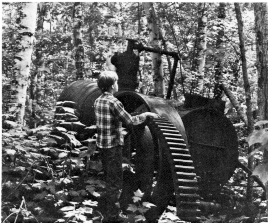
HOIST AND BOILER REMAINS at Island mine, abandoned in 1877. (Fig. 2)
