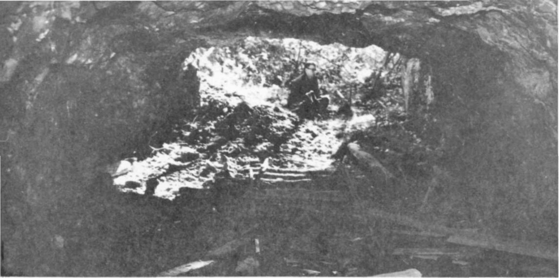
A horizontal shaft, or adit, at the Minong Mine.
