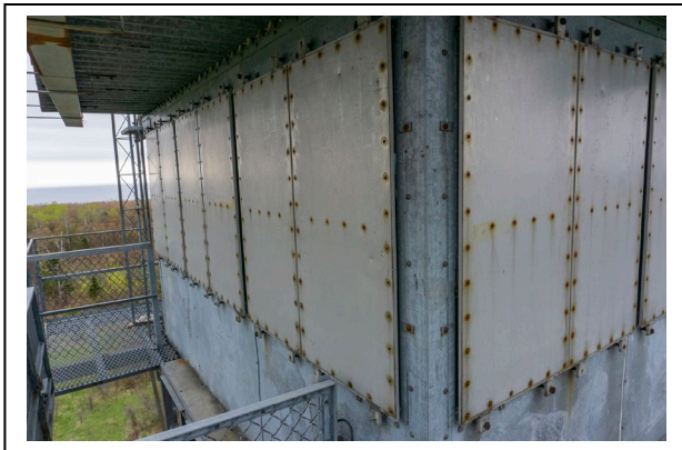
Figure 15: New Feldtmann Fire Tower cab window coverings, looking northwest. Radio antenna on balcony, left. Photo by Natalie Young, 2019.
