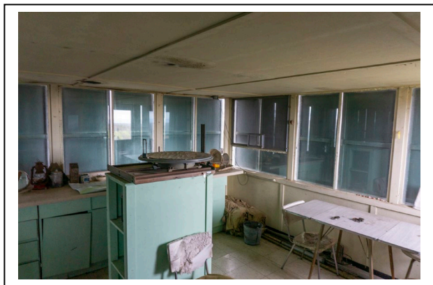
Figure 24: New Feldtmann Fire Tower cab interior, looking southeast. Fire finder in foreground. Photo by Natalie Young, 2019.
