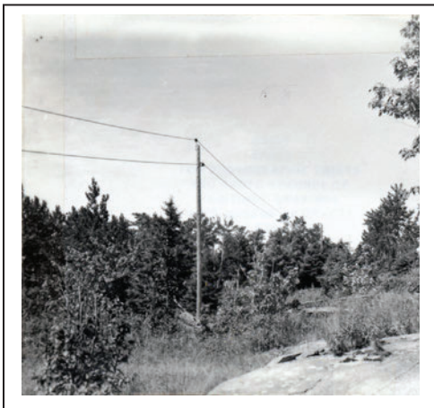
Fig. 15: Power line to Ojibway Fire Tower. Photo from National Visual Inventory Card Collection, courtesy of Isle Royale National Park, archives held at Keweenaw National Historical Park, Calumet, MI.
