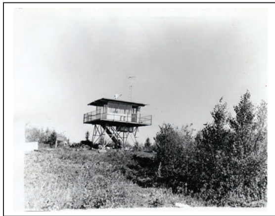
Figure 13: Ishpeming Fire Lookout Tower, 1962. Photo from National Visual Inventory Card Collection, courtesy of Isle Royale National Park, archives held at Keweenaw National Historical Park, Calumet, MI
