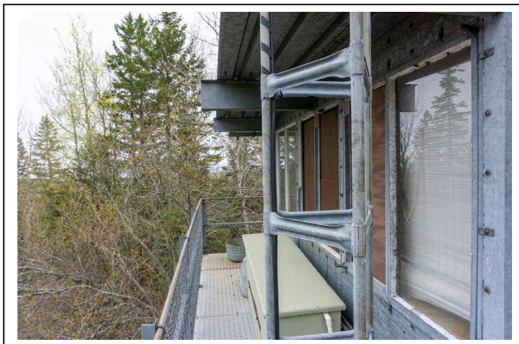
Figure 14: Water storage equipment on west side of cab, 2019, looking S. Note also plywood-covered windows. Photo by Natalie Young.
