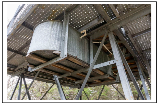
Figure 25: Corrugated metal container beneath Ishpeming Fire Tower cab floor, 2019, facing SW. Photo by Natalie Young.
