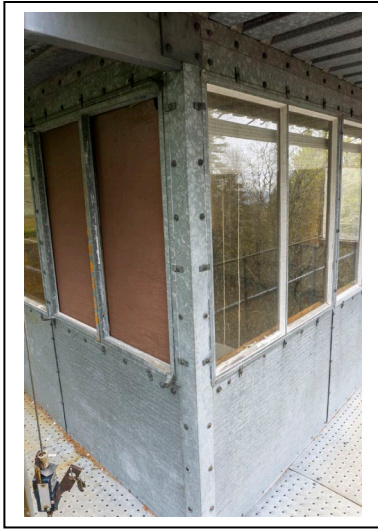
Figure 15: Southwest corner of Ishpeming Fire Tower cab, 2019, facing NE, showing plywood window coverings on west side. Photo by Natalie Young.
