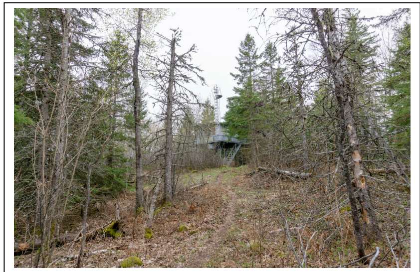
Figure 3: Ishpeming Fire Tower, 2019, looking SW. Photo by Natalie Young.
