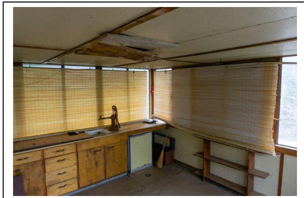
Figure 20: Showing hand pump at sink for water and poor condition of ceiling on interior of Ishpeming Fire Tower cab, 2019, looking NE. Photo by Natalie Young.
