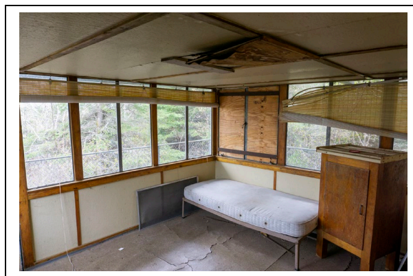
Figure 23: Ishpeming Fire Tower cab interior, 2019, looking SW. Photo by Natalie Young.
