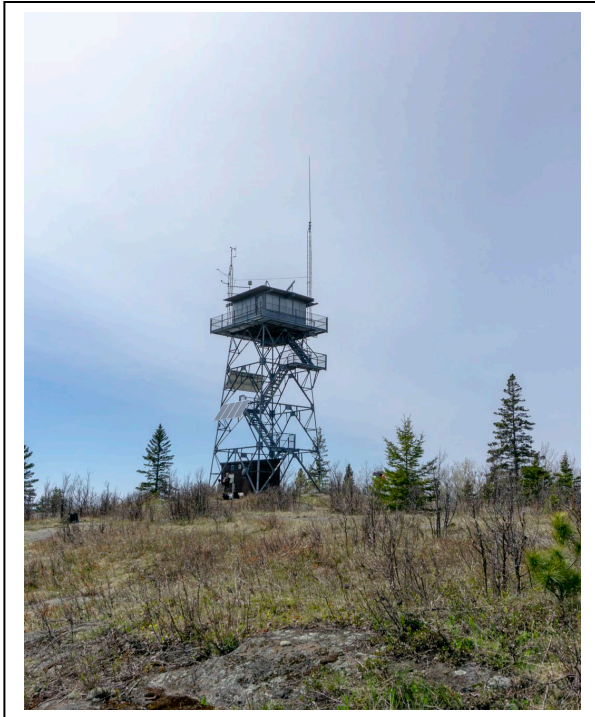
Figure 2: Ojibway Fire Tower, 2019, looking northwest. Photo by Natalie Young.
