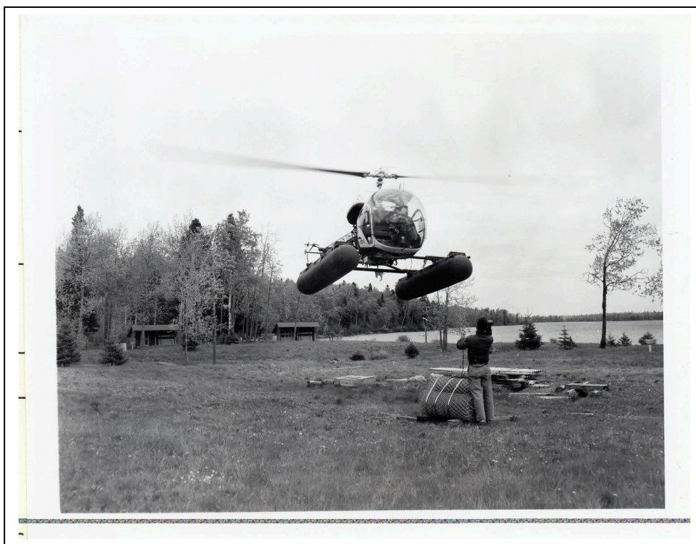
Figure 42: Helicopter transporting bundles of construction materials from the Daisy Farm campsite staging area to the Ojibway Fire Tower construction site, July 1964. Image from National Visual Inventory Card collection in Isle Royale National Park archives held at Keweenaw National Historical Park, Calumet, MI.
