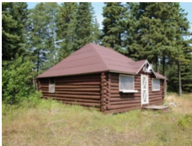
View of the Anderson/Scotland Cabin
