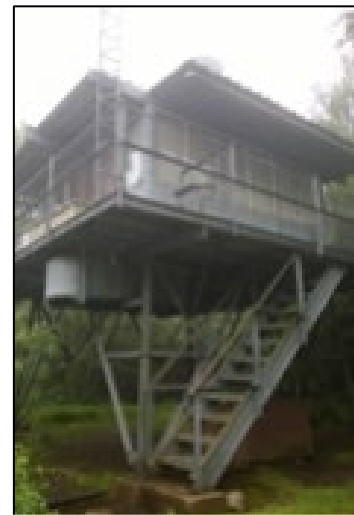
View of Ishpeming Fire Tower and associated equipment
