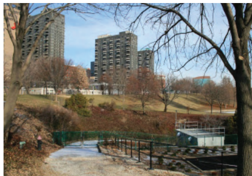
Service road to heating, ventilating, and air conditioning systems.
