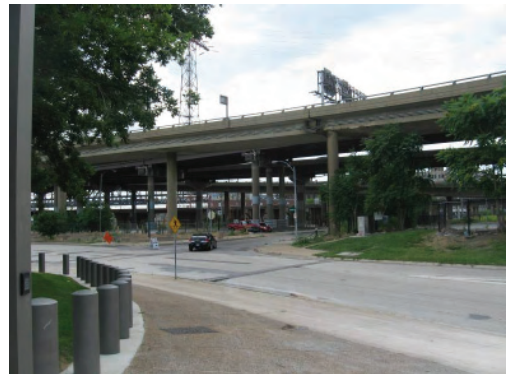
Poplar Street, beneath the Poplar Street Bridge.
