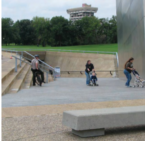
Concrete steps and granite ramps leading to the underground visitor center.
