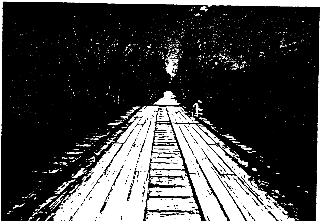
Bridge of the Shell Road/Old Road/Christmas Plantation Headquarters Road, looking NE from west bank of Bayou des Familles. 3/86.
