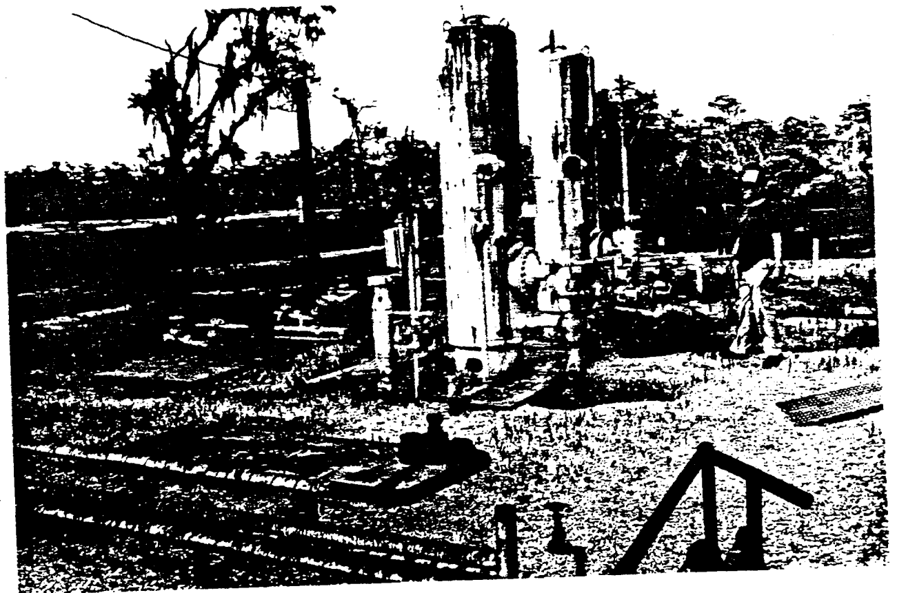
Barataria Oil Field, showing separator tanks on concrete pads and flow lines. 4/86.
