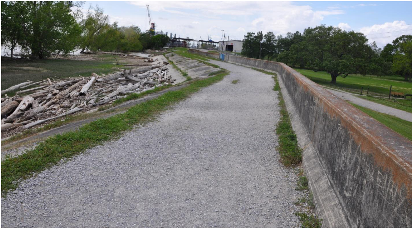
Figure 31. Photograph of fortified wall at the Chalmette Unit. The Chalmette Unit of the park is on a natural levee complex of Mississippi River meander belt 1 (Hml1). An artificial levee was built atop the natural levee, and a fortified wall was constructed atop the artificial levee. The wall runs through Chalmette Battlefield. The wood debris along the levee was deposited there during high water levels on the river. Photograph from Peek (2017, figure 10).
