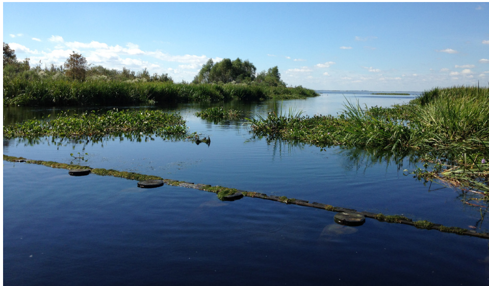
Figure 35. Photographs of the eastern shoreline of Lake Salvador. To reduce the risk of breaching between the eroding eastern shoreline of Lake Salvador into the Bayou Segnette Waterway, an earthen dike was built in 1996 and filled to reestablish the marsh. This project area is generally known as the geo-crib. In the top photograph: The straight Bayou Segnette Waterway is on the left. Lake Salvador is on right. The dike runs down the side of the canal, and the geo-crib is offshore and ties into additional rock-shoreline protection extending out of the frame of the photograph to the right. In the bottom photograph: A wooden bulkhead at the Tenneco canal originally dead-ended at a drilling location in the marsh until the lake eroded into it. Photograph [top] from USACE (1998). NPS photograph [bottom] by Courtney Schupp (NPS Geologic Resources Division), taken looking westward into Lake Salvador on 28 October 2015.
