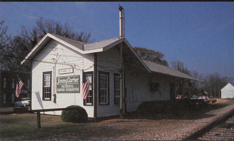
Plains Depot Main Street and South Hudson Street. The depot was completed in 1888 after the town called the Plains of Dura moved a short distance southward to take advantage of the new railroad line and shortened its name. In 1919, 66 carloads of hogs and cows were shipped from the depot; 6,000 to 10,000 bales of cotton were shipped annually from Plains in the 1920s. The building is restored as Carter's 1976 campaign headquarters and has served as the National Park Service visitor center.
