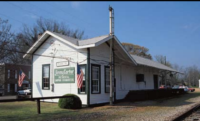
PLAINS DEPOT Main and South Hudson streets. The depot was completed in 1888. The town, then named Plains of Dura, moved a short distance south to take advantage of the new railroad line and shortened its name to Plains. In 1919, 66 carloads of hogs and cows were shipped from the depot. In the 1920s, 6,000 to 10,000 bales of cotton were shipped annually from Plains. The building has been restored to its 1976 appearance as Carter's campaign headquarters.
