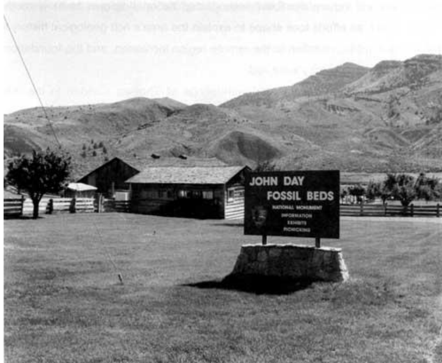
Headquarters, John Day Fossil Beds National Monument, Sheep Rock Unit. Photo courtesy NPS.
