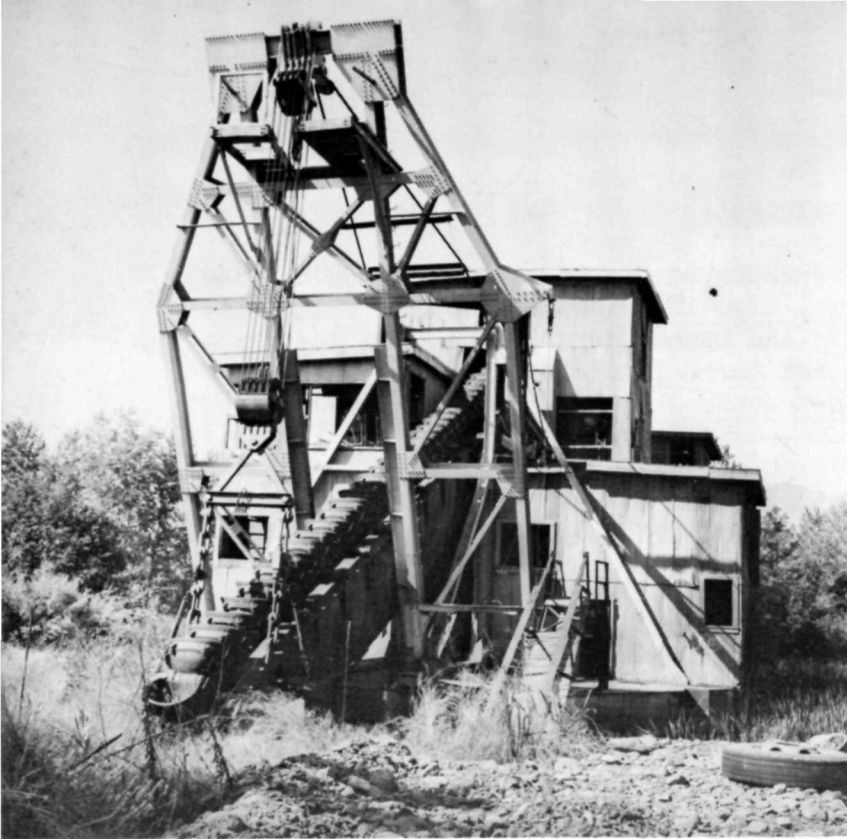
Gold mining dredge at Mount Vernon. Used as recently as 1946, it is nearly intact and could be of interest to tourists.
