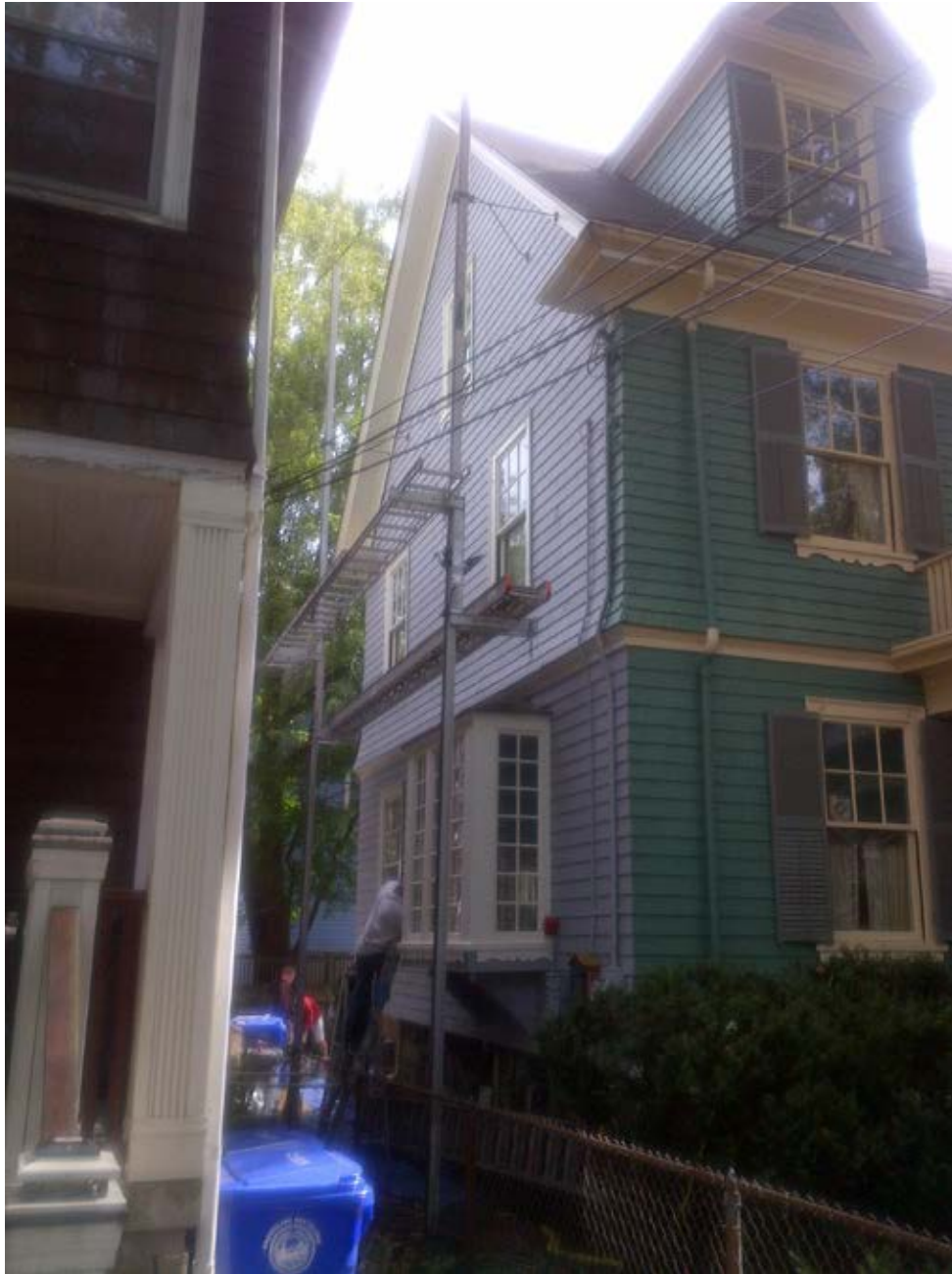
Figure 15. House repainted. JOFI uncatalogued collections. NPS, 2012.
