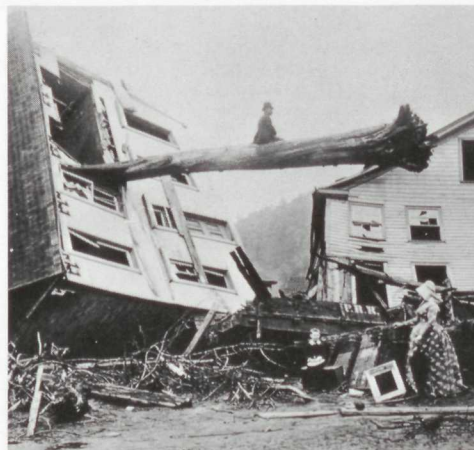
The flood snapped large trees like sticks and turned them into battering rams that could pierce walls.
