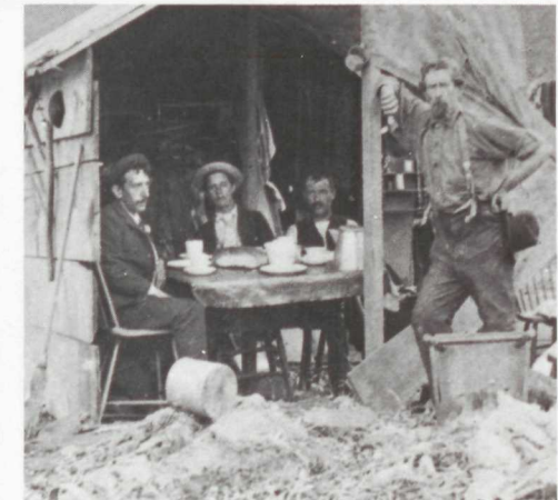
Survivors lived in army tents and lean-tos. Prefabricated "Oklahoma" houses, furnished with essentials, were later sold for $250.
