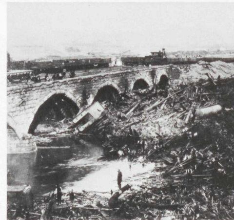
A jam at stone bridge caused a 10- to 30-foot lake over Johnstown. The fire there, probably caused by oil and hot coals, burned for 2 days.
