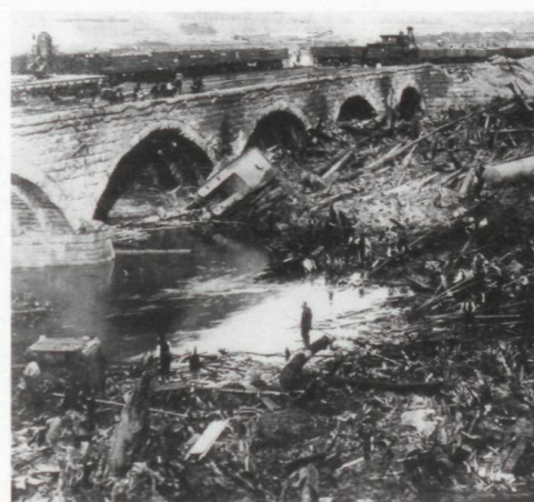
A jam at stone bridge caused a 10- to 30-foot lake over Johnstown. The fire caused by oil and hot coals burned for two days. More than 80 people died here.
