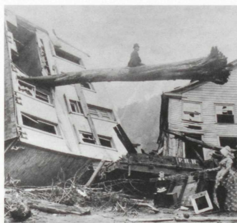
The flood snapped large trees like sticks and turned them into battering rams that pierced walls.
