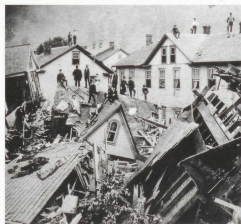
Shattered buildings were thrown into jumbled piles three stories high, completely filling some blocks.
