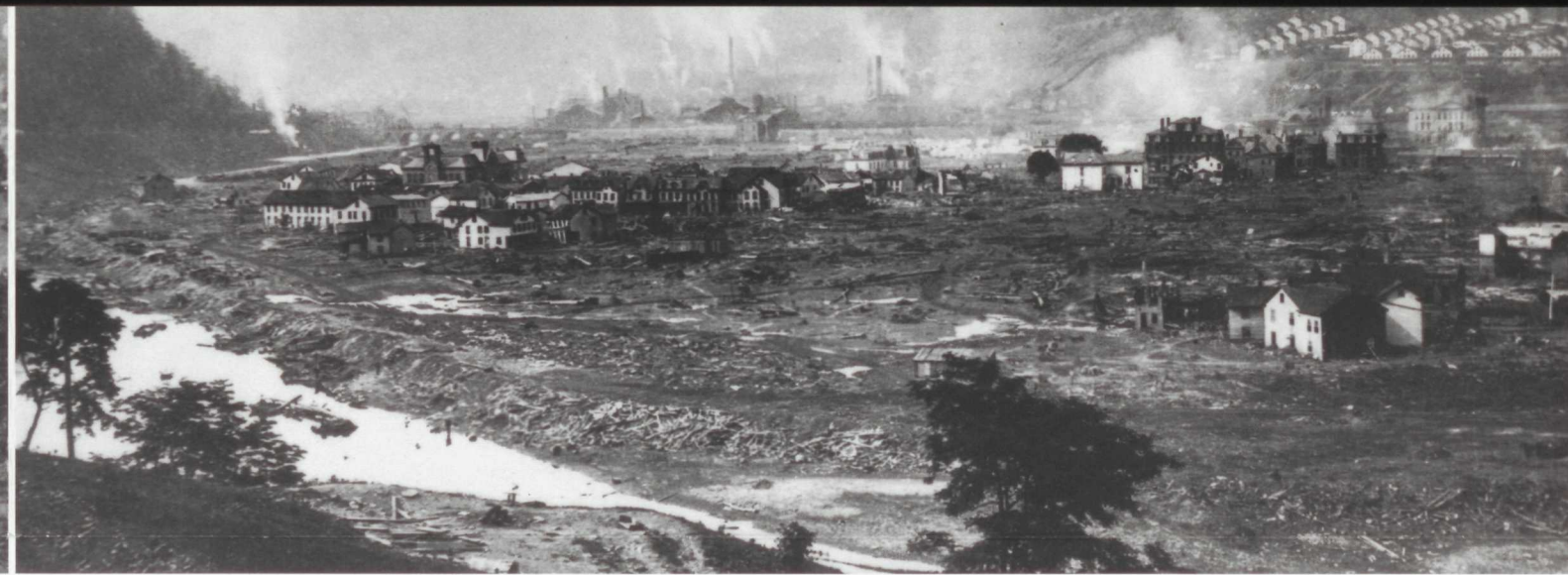
The wave reduced the area to rubble in 10 minutes. Some buildings were spared where the waves split.
