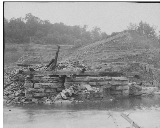
View of the north dam abutment and spillway in 2007(left photo). Photo by NPS staff. The sluice gate remains of the South Fork Dam, taken after the May 31, 1889 break (right photo). Photo courtesy of JAHA
