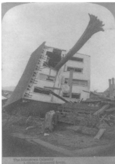
FIGURE 14: George Barker, The Johnstown Calamity: A Slightly Damaged House , one half of stereograph card. (Prints & Photographs Division, Library of Congress, 3447000).
