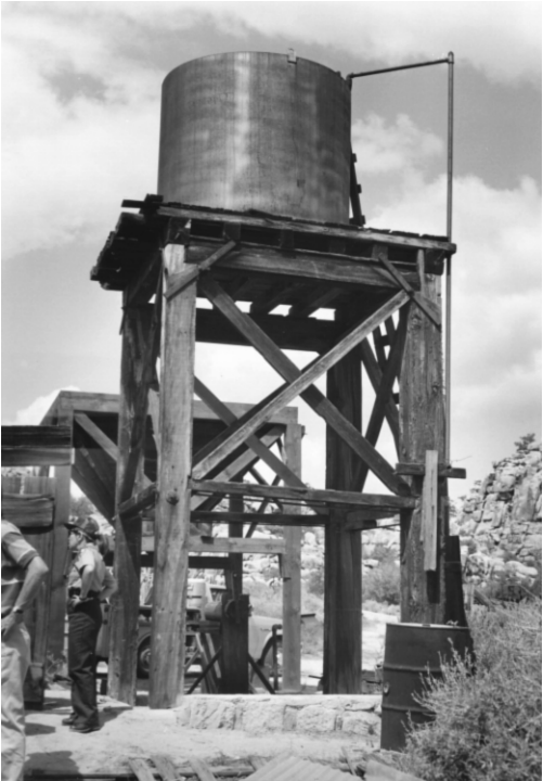
Buildings and Structures #5: Desert Queen Ranch water tower, looking northwest. (PGSO, LCS, 1992)
