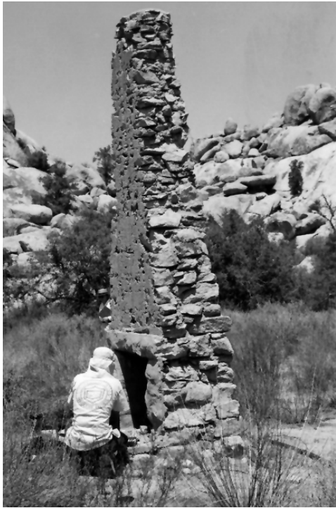
Buildings and Structures #12: Cow Camp chimney, looking north. (PGSO, LCS, 1992)
