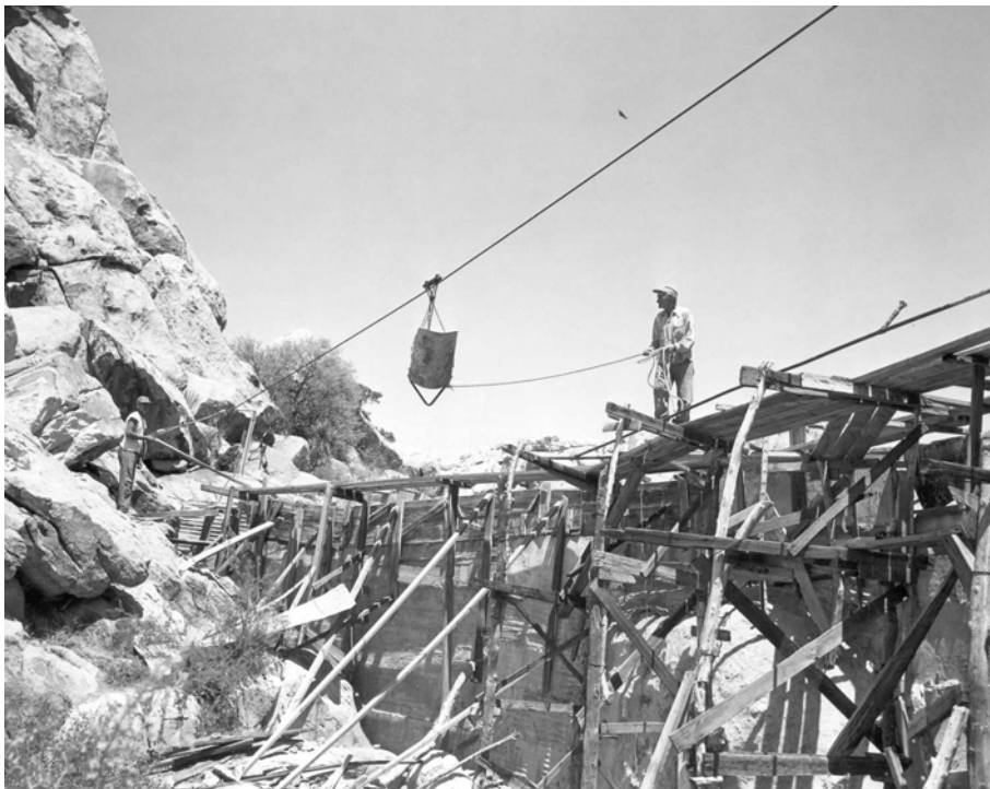
Buildings and Structures #9: Desert Queen Ranch, construction of reservoir dam, looking north. (Joshua Tree National Park archives, accession #693-124, ca. 1940)
