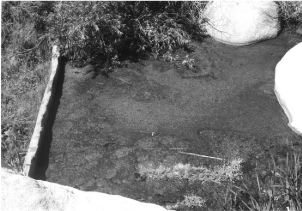
Buildings and Structures #16: Barker Dam catchment basin, looking northwest. (PGSO, LCS, 1992)
