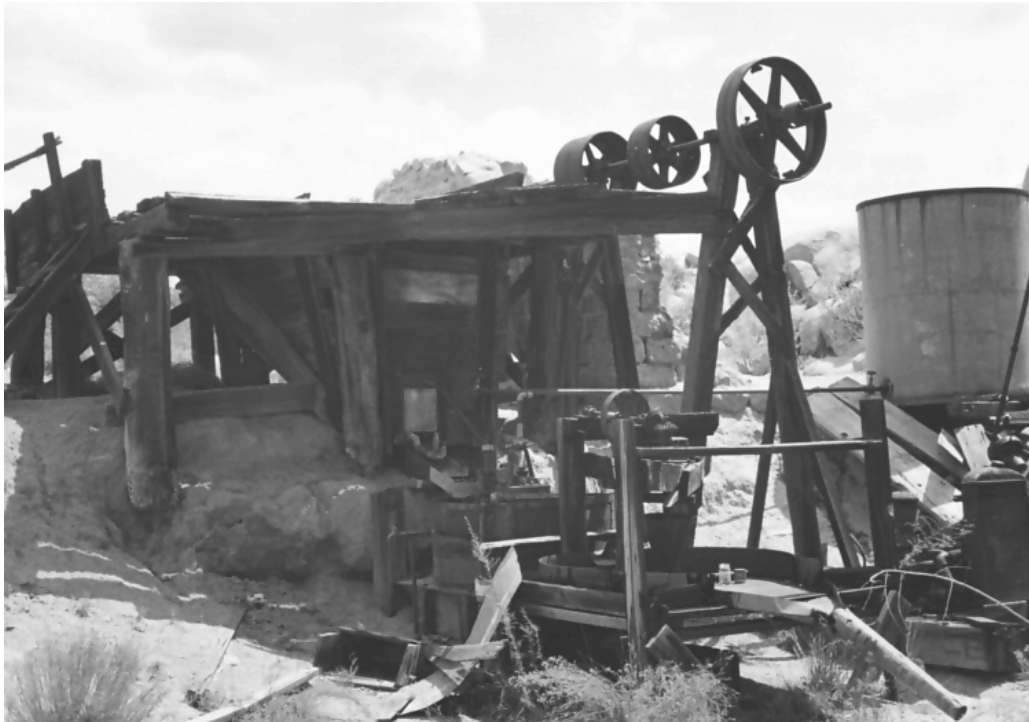
Buildings and Structures #8: Desert Queen Ranch huntington mill, looking southeast. (PGSO, LCS, 1992)
