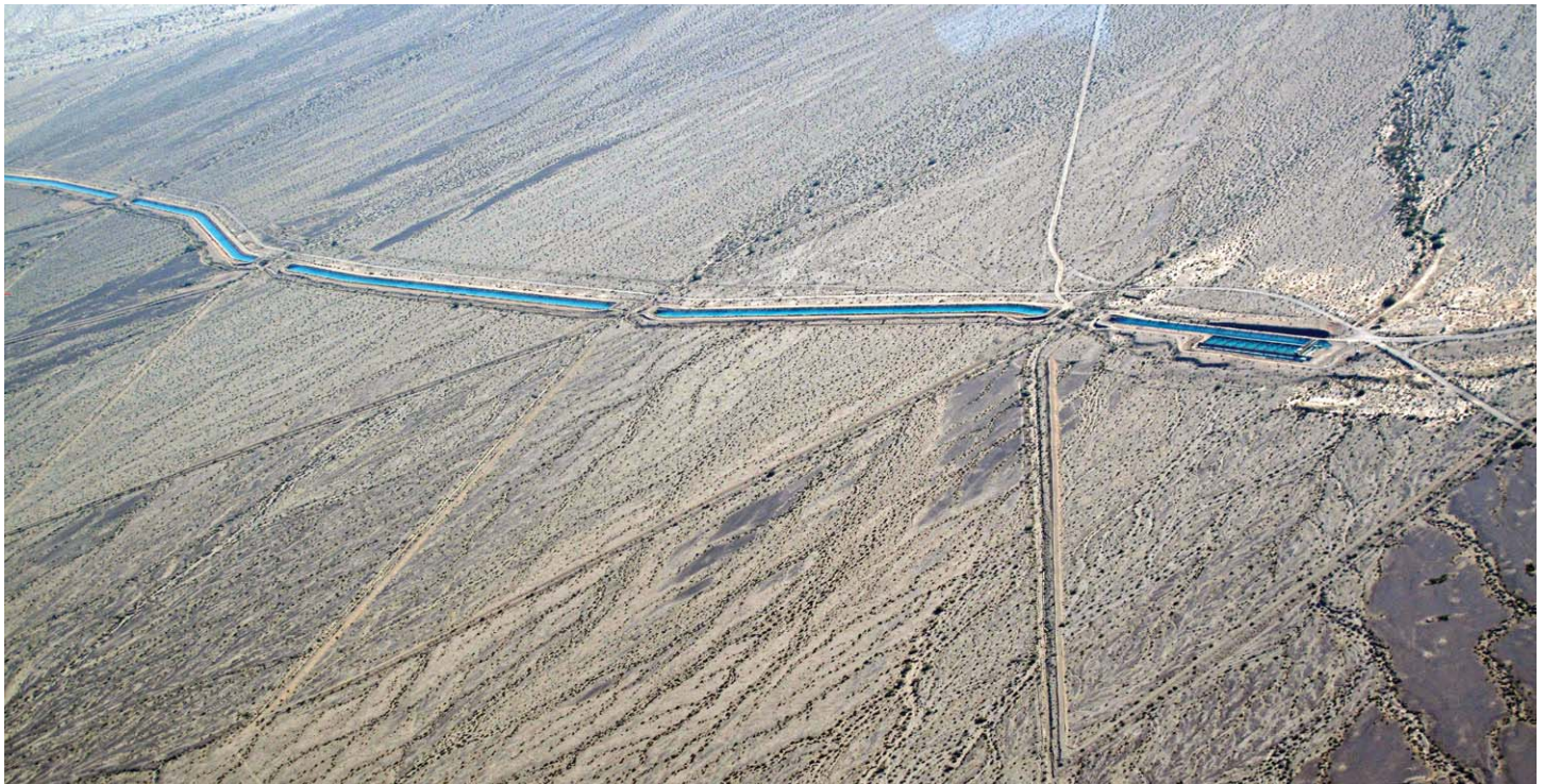
The Colorado River Aqueduct as it transitions from canal to tunnel. The aqueduct forms the eastern edge of the study area. Photo by Ecoflight, 2011.
