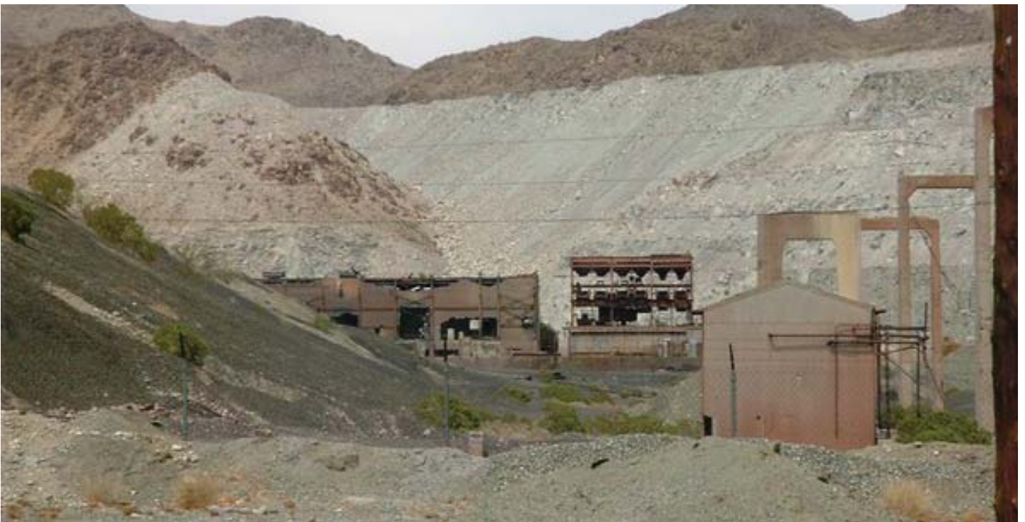
Remnants of processing facilities at Eagle Mountain Mine (2002). Photo courtesy of Roy Hooper.
