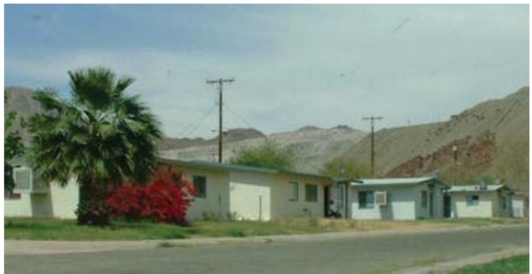
In contrast, occupied homes directly across the street area (2002). Photo courtesy of Roy Hooper.
