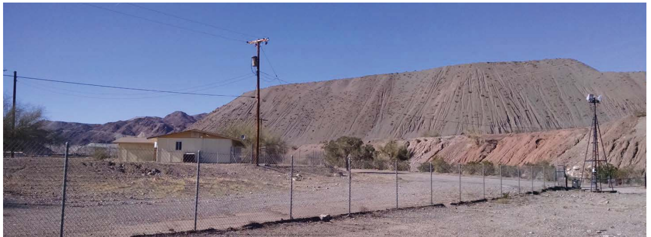
Aggregate and other rock products continue to be extracted from tailing piles at the Eagle Mountain Mine
