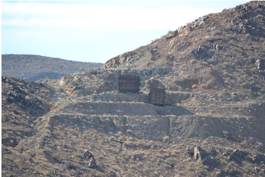
Figure 1: Tipples (ore bins) at the Silver Bell Mine site as seen from Pinto Basin Road, looking south to the Hexie Mountains, Joshua Tree National Park, 2016
