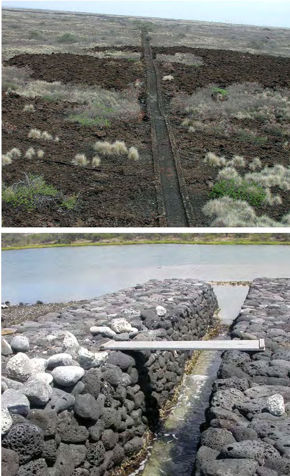
Figure 17. The cultural resources of Kaloko-Honokōhau National Historical Park are deeply connected to the park's geology. Māmalahoa trail (top) crosses lava flows in the park. A fishpond makaha (sluice gate; bottom)—constructed from basalt boulders—allows for water exchange with the pond and prevents larger fish from escaping. National Park Service photographs. Trail photograph courtesy Jon Jokiel (Kaloko-Honokohau National Historical Park). Makaha photograph by Rebecca Beavers (NPS Geologic Resources Division), available online: http://www.nature.nps.gov/geology/cfprojects/photodb/Photo_Detail.cfm?PhotoID=668 . Accessed 13 May 2011.
