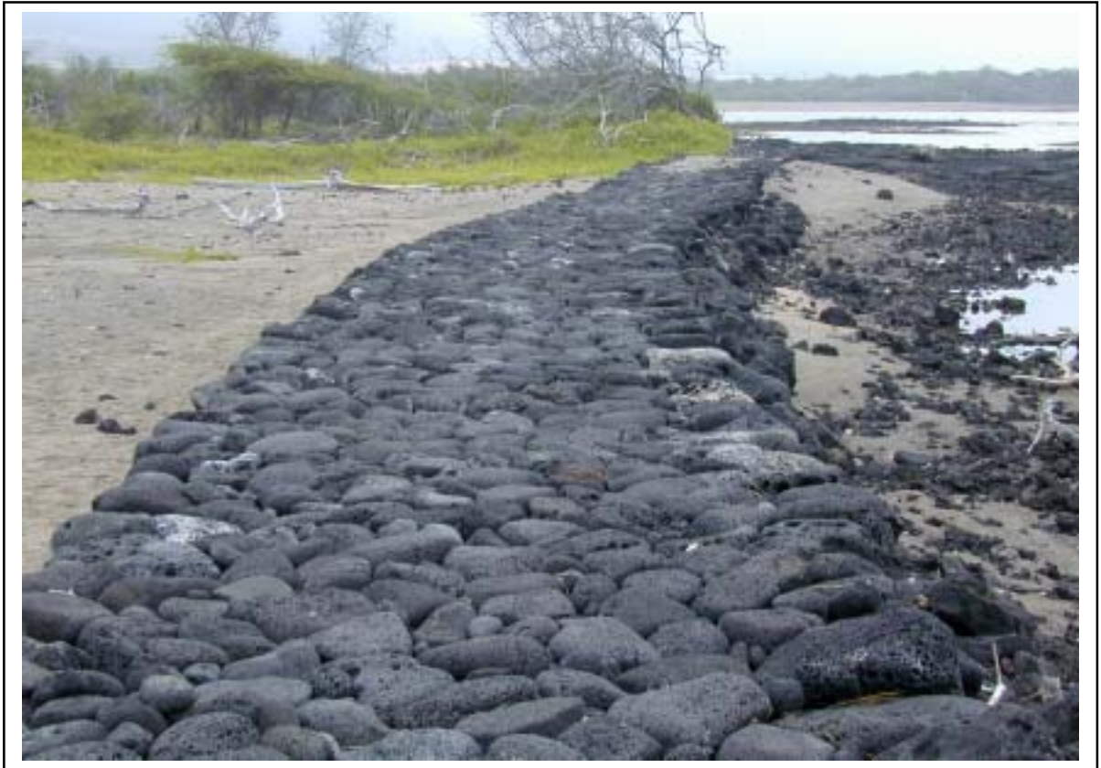
Access wall on shore of Honokōhau Nui (area formerly a part of the 'Aimakapā Pond Complex (KPA Photo No. 1333)
