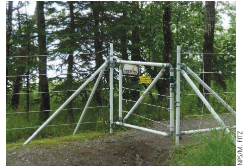
Brooks Camp Campground is surrounded by an electric fence. It is bear-resistant, but not bear-proof. Campers must take precautions so that bears are not tempted to enter the campground.
