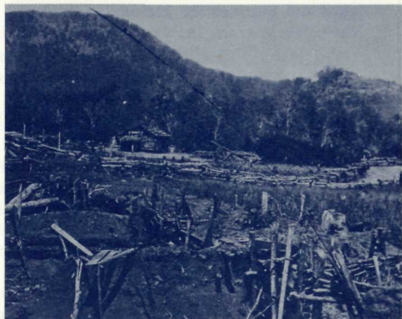
Federal earthworks on a farm at the base of Little Kennesaw.
