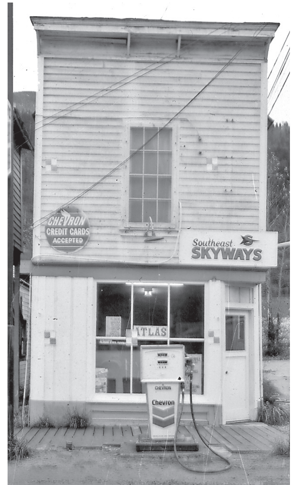
Verbauwhede's Cigar Store, as it appeared prior to National Park Service restoration, March, 1981
