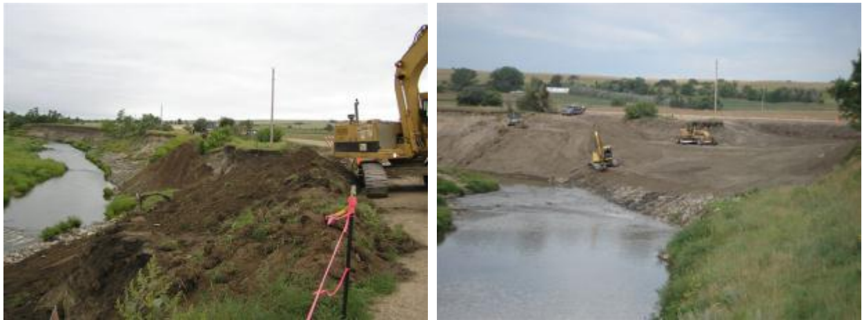
Figure 7. Photos of riverbank repair along Taylor's Bluff in KNRI, August 2009. On the left, Taylor's Bluff prior to major excavation, fill, and rip rap installation; on the right, Taylor's Bluff in the process of rip-rap installation.
