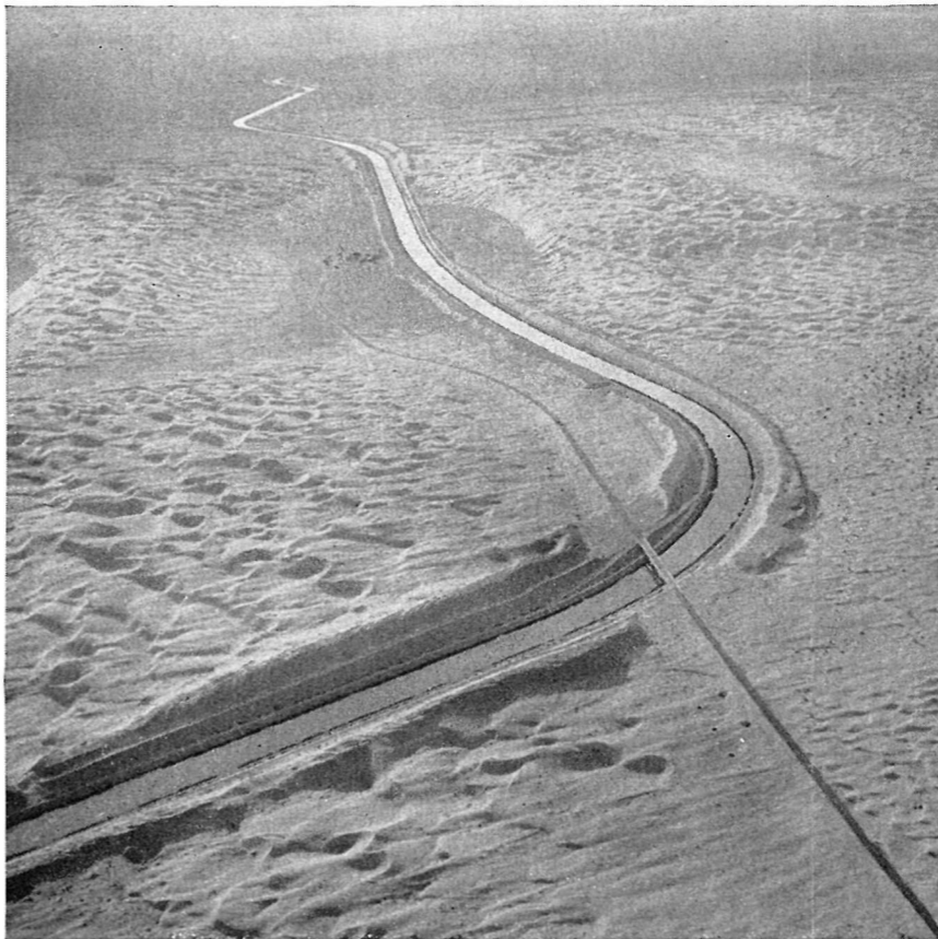
All-American Canal winds through sand hills
