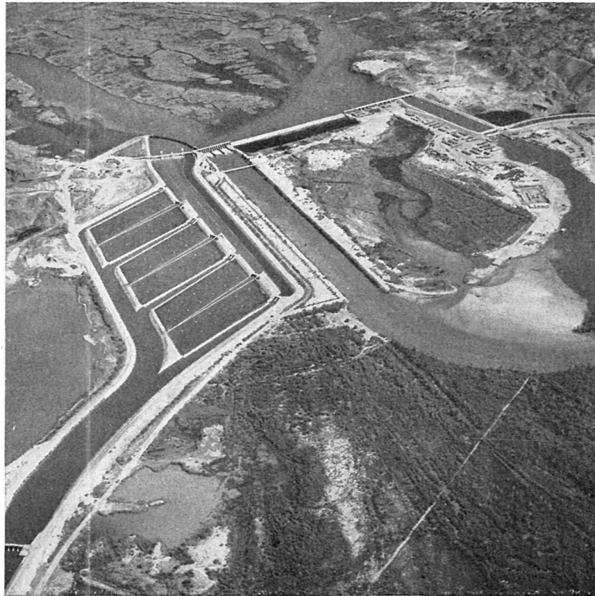
Imperial Dam and desilting works
