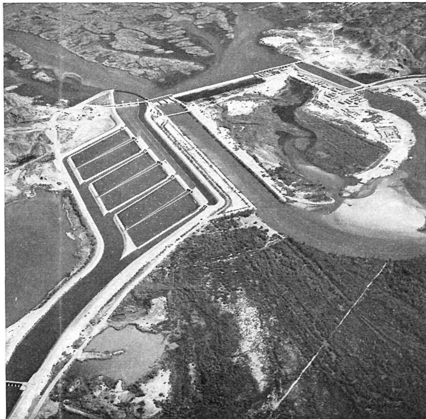
Imperial Dam and desilting works
