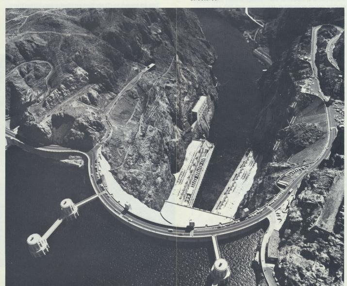
The reservoir, Lake Mead, is America's largest man-made reservoir. Named for Dr. Elwood Mead, Reclamation Commissioner during Hoover's construction, the lake backs up 110 miles behind the dam and is capable of storing 28.5 million acre-feet of water. (An acre-foot of water is 325,851 gallons, or enough to cover an acre to a depth of one foot.)
