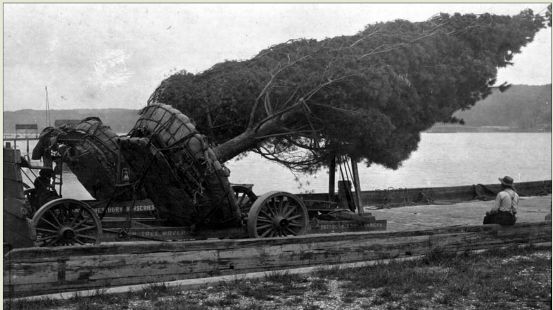
Mature trees ready for transporting by barge, c. 1900.
