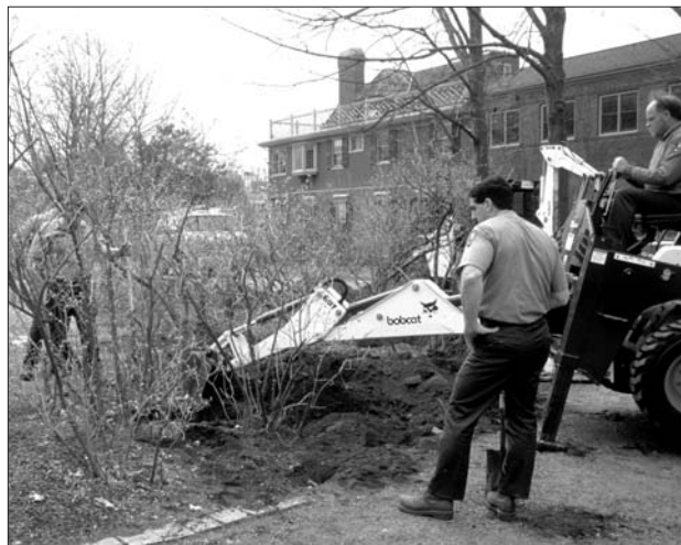
Use of a backhoe to remove a tree stump can cause significant site disturbance and should be used only in locations where adjacent resources can be well protected.
