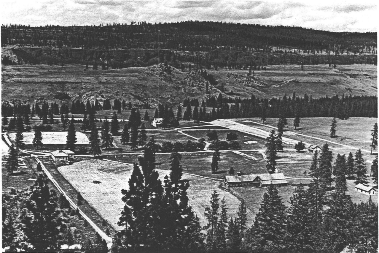
G. Historic Fort Spokane ca. 1940, northeast corner. The guardhouse, quartermasters and two officers' quarters are visible.
