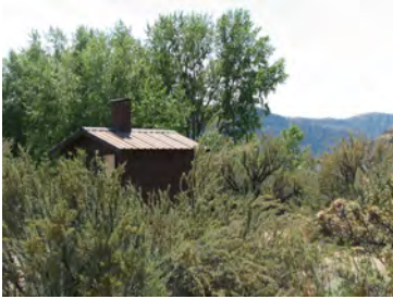
Vault toilet at Keller Ferry
