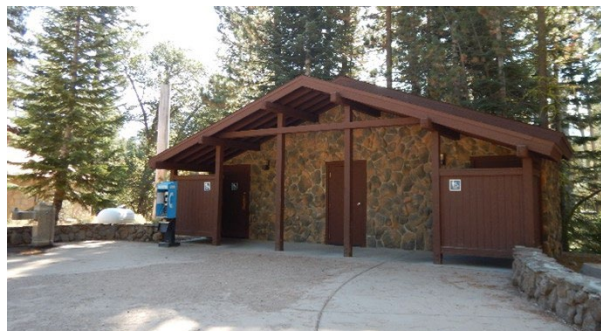
FIGURE 6. LOOMIS PLAZA RESTROOMS BUILDING
