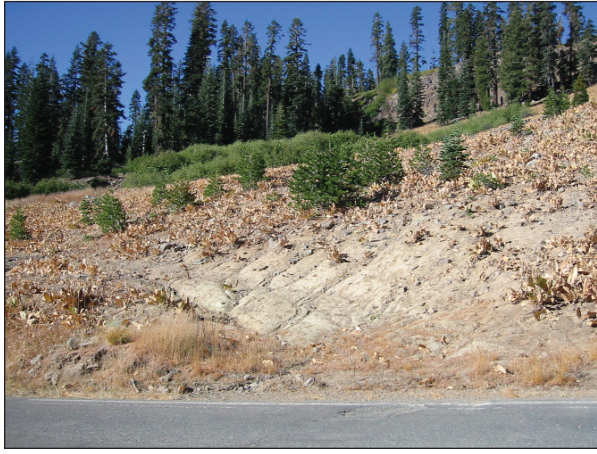
Erosion along the old service road where it connects with the Park Road
