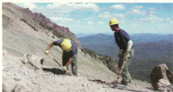
Park trail crew at work on the Lassen Peak trail
