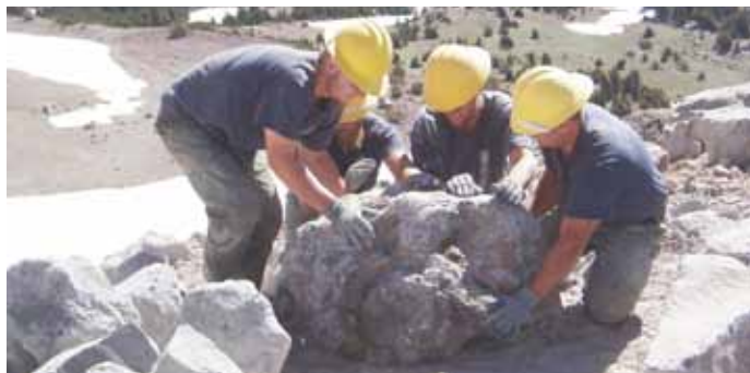
Park trail crew at work on the Lassen Peak trail
