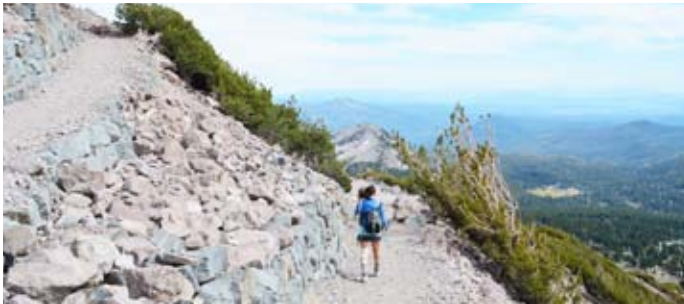
A hiker passes through switchbacks with new rock retaining walls
