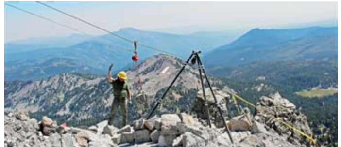
A trail crew member guides a boulder on a cable and pulley system
