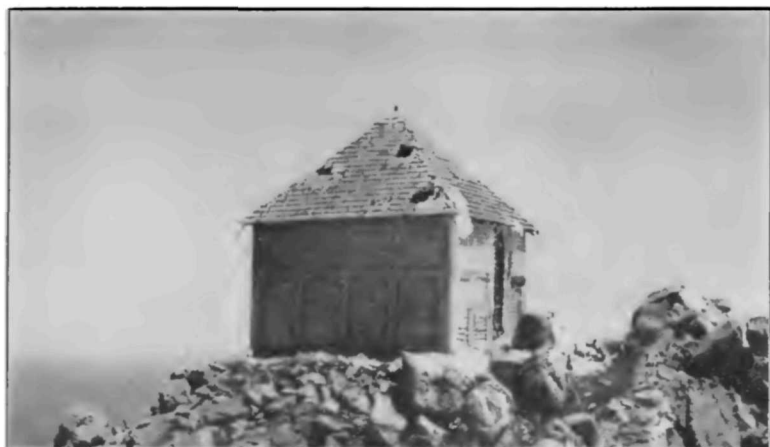
FIG. 5. THE FIRE LOOKOUT STATION OF THE U. S. FOREST SERVICE ON JUNE 26, 1914. The holes in the roof were probably made during the eruption of June 14. The house has been entirely destroyed by later eruptions.
