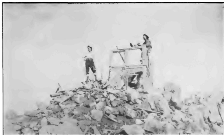
FIG. 6. THE LOOKOUT STATION AS SEEN ON OCTOBER 7.
