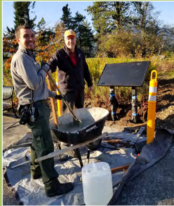
Bonneville Lock and Dam Natural Resource Specialist, Ranger Mason Scharfe and Volunteer Bill Eber install a new base for the updated Lewis and Clark interpretive wayside exhibit. Photo courtesy of US Army Corps of Engineers.
